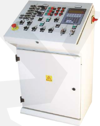
Operating Console Type Panels
